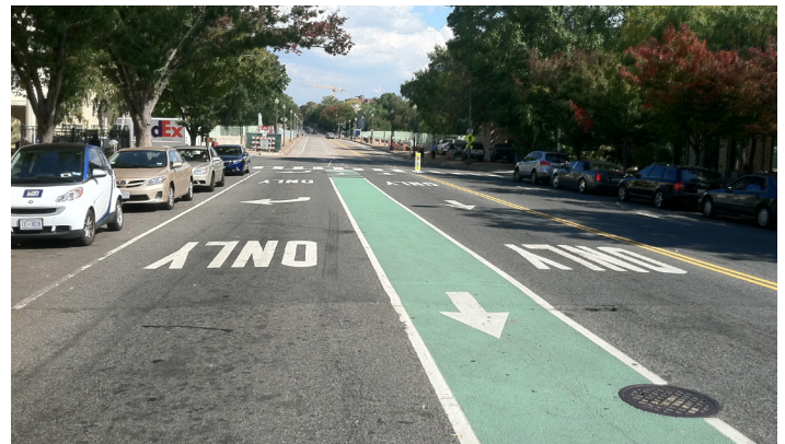
Green paint used to make a conventional bicycle lane more visible.
