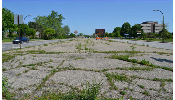
Concrete medians dominate the landscape in Area 2
